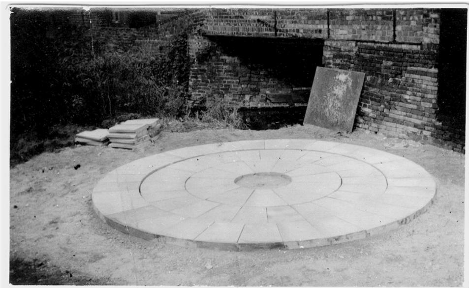
This photo was given to me as a memento when I left Harris and Pearson for the R.A.F. It shows a setting out of the bottom course of a Blast Furnace “bosh” and I was told that it is one of the last if not the last to be made at H&P from local clay. This is quite probable, since clay based blast furnace bosh brick were rapidly going out of fashion, being replaced by basics such as carbon or graphite.
